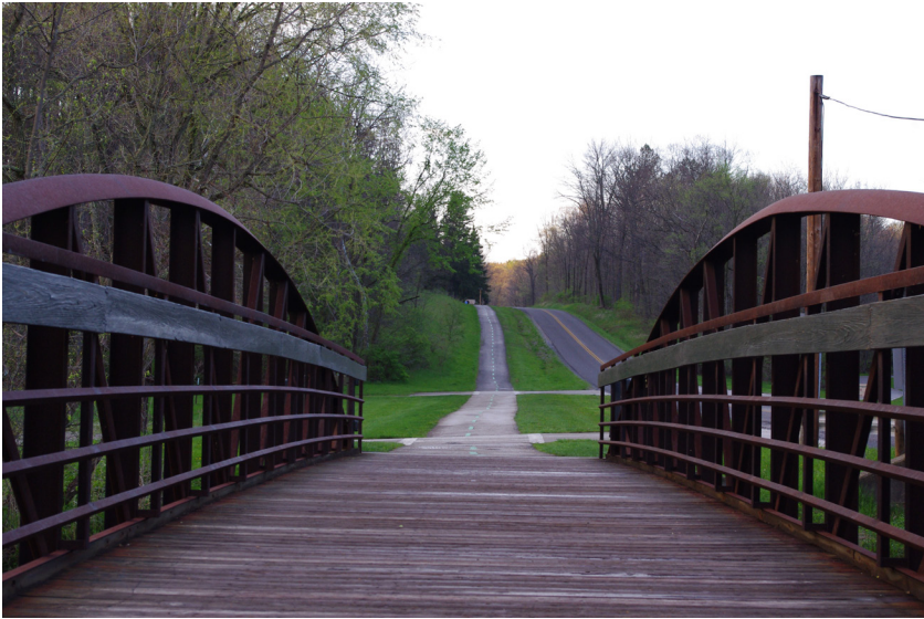
Figure 3: Bridge and Trail
